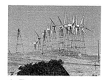
▲ The blades of a modern windmill act like a turbine. Wind energy turns the turbine, which turns a drive shaft, which turns a magnet inside the built-in generator.
